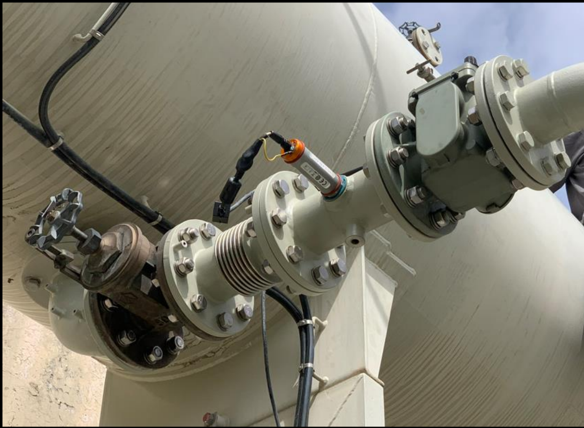
Mounting on the pipeline
